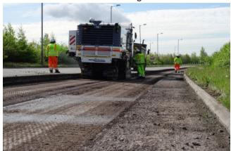
The plant / machinery has continued planing out to a depth of 270mm. This week over 4000 tonnes of planings have been transported off site.
